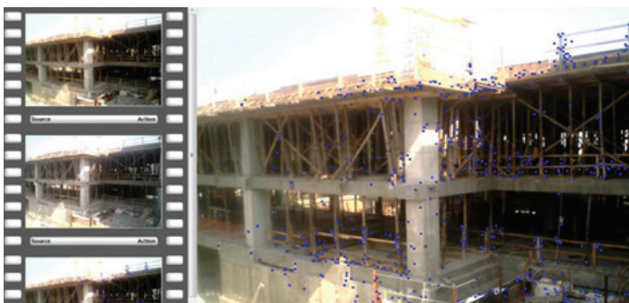
Faculty and students in the School of Civil and Environmental Engineering, with support from the National Science Foundation, are developing a new 3D imaging system that provides data on the condition of infrastructure more accurately and cost-effectively than existing technology. Private support through industry partnerships will further enhance this advanced research.
